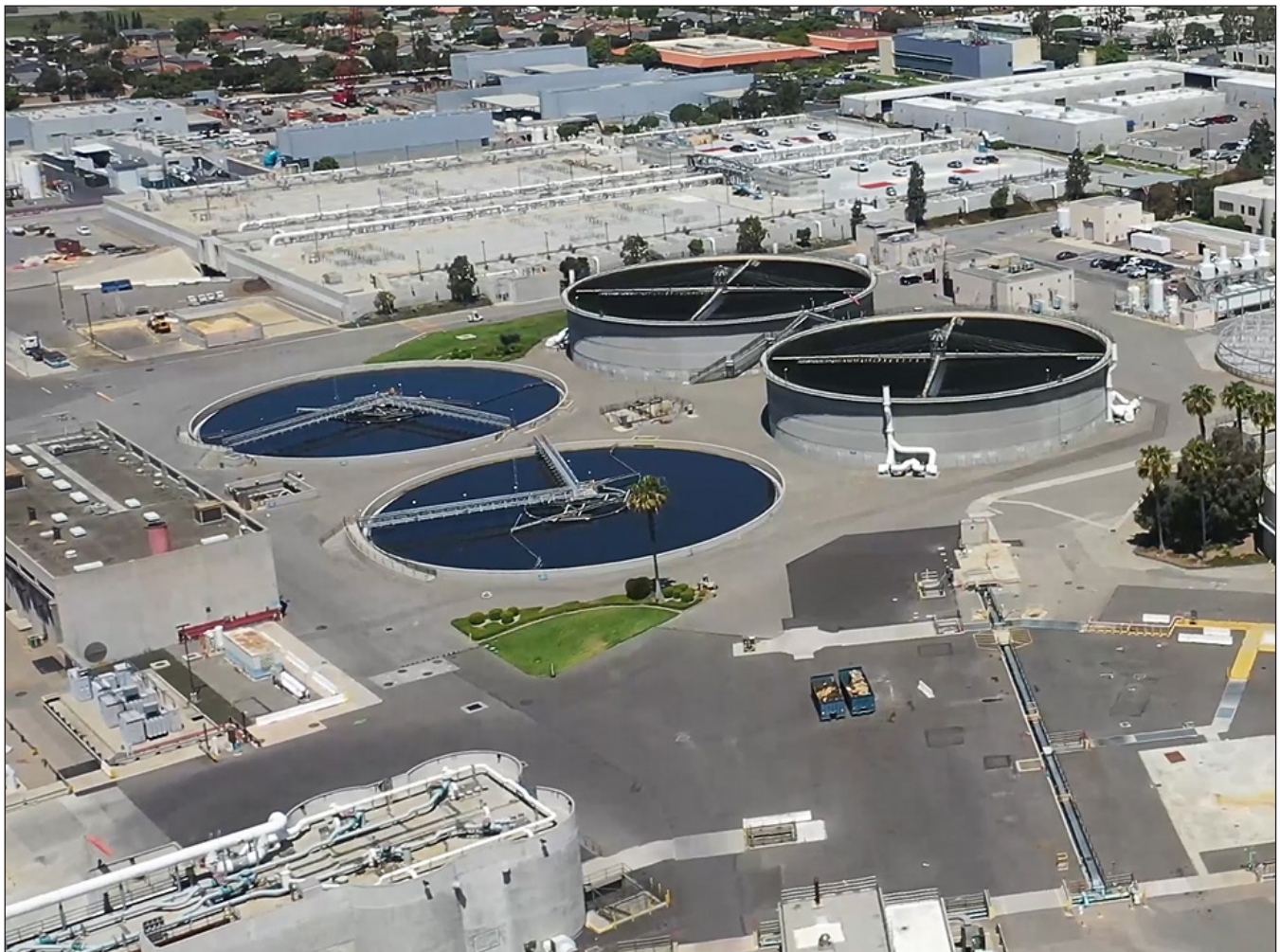
Reclamation Plant No. 1 in Fountain Valley.
