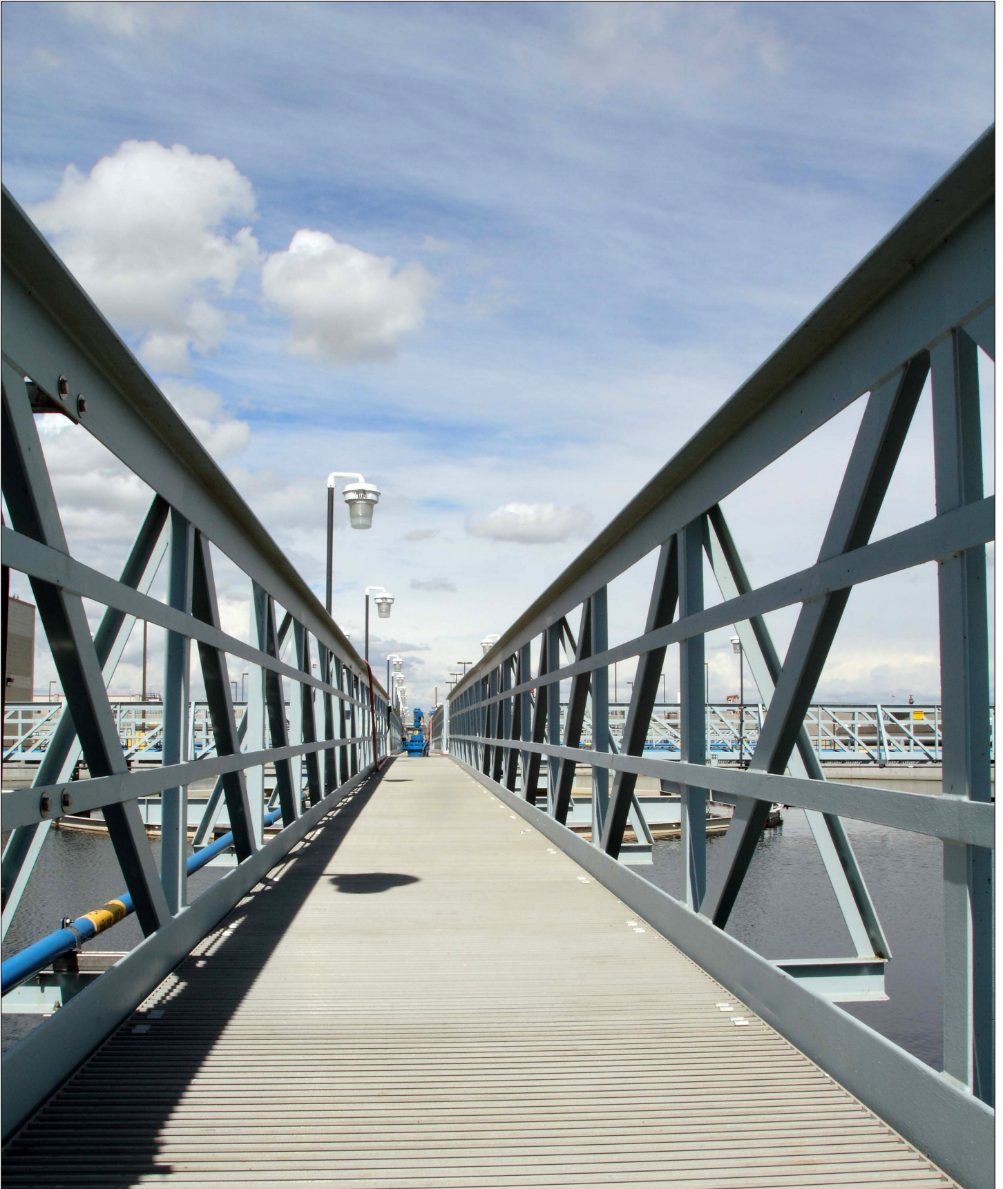
Secondary clarifier at Plant No. 1 in Fountain Valley.
